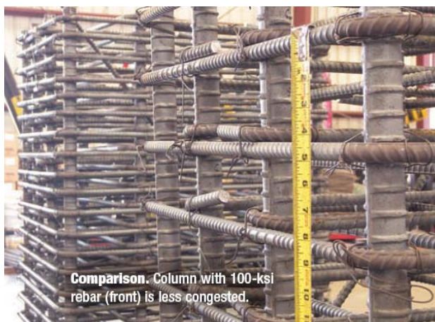
Figure 9: Physical column congestion comparison (source: courtesy of Harris Rebar)
