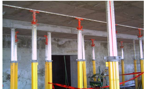
Figure 12: Drop head at slab soffit (source: courtesy of CKC)
