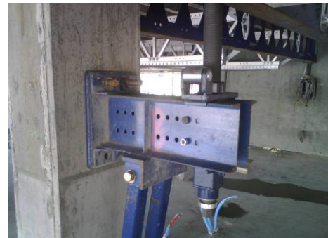
Figure 6: Column-hung forming system (source: courtesy of CKC)
