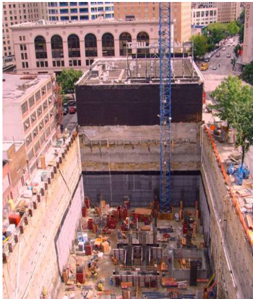
Figure 5: Escala foundation mat, Seattle, WA (source: courtesy of JE Dunn)
