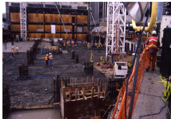
Figure 2: Metropolitan Tower foundation pour, Seattle, WA (source: courtesy of CKC)
