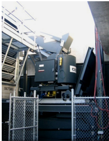
Photograph 6-6 BMU Stored Below Roof to Eliminate Silhouette
