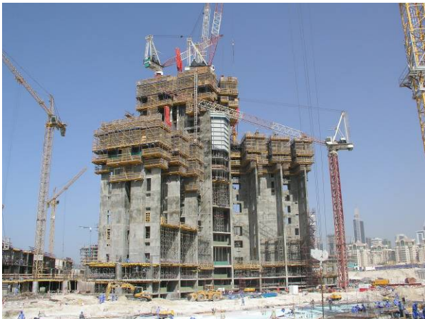
Figure 23 – Self-Climbing Formwork System
