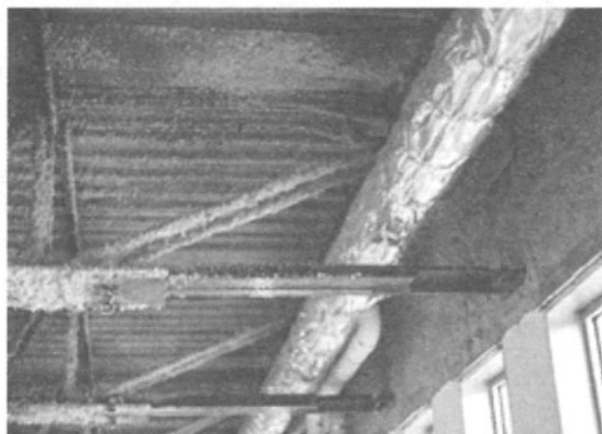
Photo 4 Fire protection of floor truss
