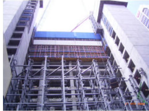
View of lift frame grillage from Phillip Street
