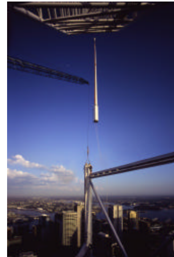
Erection of north western mast
