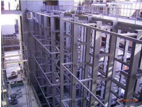
View of lift frame grillage from the atrium
