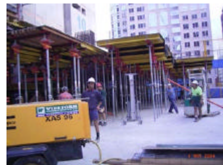
Typical floor formwork table arrangement
