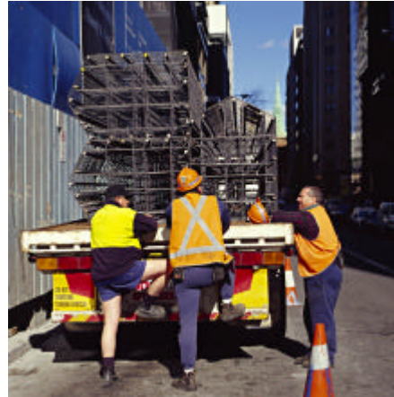
Prefabricated column cages
