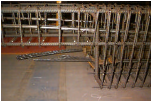
Sample prefabricated typical floor beam cage
