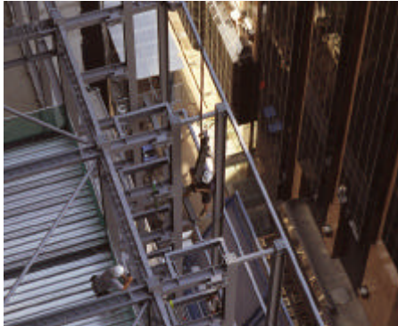
View of partially erected lift frame
