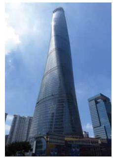
Figure 14. The Shanghai Tower's double façade system adds a lightness and complexity of geometry through its structural layering. © Tansri Muliani
