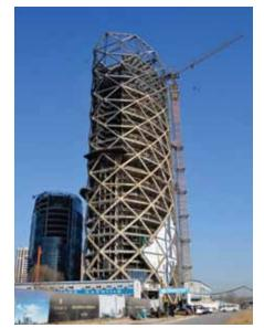
Figure 11. The Poly International Plaza, Beijing, employs a diagrid system using concrete-filled tubes that vary in diameter and thickness from  $\emptyset$ 1.3 m, 50 mm thickness at the base to  $\emptyset$ 0.7 m, 20 mm thickness at the top. Alternate floors are connected to the diagrid to create tensile connections between the nodes. Intermediate floors are hung from the floor above.
