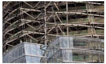
Figure 8. The double-façade system of the Shanghai Tower. The system encloses multi story atrium spaces that sit outside of the primary structural system, which is composed of megacolumns combined with outrigger floors.
