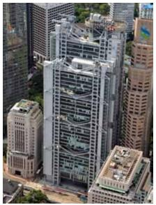
Figure 9. In 1985 the Hong Kong and Shanghai Bank by Foster + Partners launched the use of highly expressive structure and prefabricated components into the realm of tall building design.
