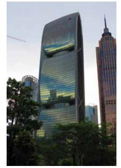
Figure 4. Pearl River Tower, Guangzhou uses its sculpted form to direct wind toward turbines situated at the recesses in the façade. © Tansri Muliani
