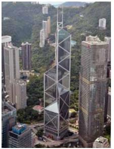
Figure 10. The use of the diagonal as a form-giving device transforms the Bank of China into an iconic tower that is visually distinct from the surrounding, more traditional skyscrapers in Hong Kong.
