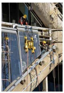
Figure 13. Workers install the glazing that will form the double façade system on the Poly International Plaza. The coordination of such complex geometries is possible only through the advancements of BIM systems.
