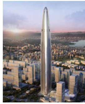
Figure 5. Wuhan Greenland Center's distinctive floor slots help to reduce the vortex shedding. © AS + GG Architects
