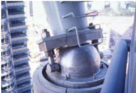
Figure 7. Bridge leg bearing.
