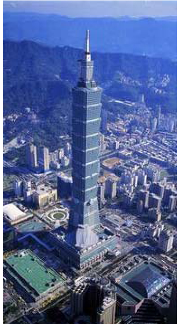
Figure 8. Taipei 101 shows tapering modules. Credit: Dugald Mackay courtesy C. Y. Lee & Associates.
