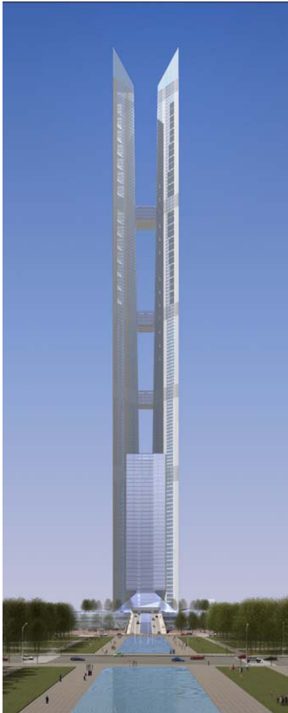
Figure 12. Incheon 151 in South Korea uses slots to disrupt vortex formation. Credit: John Portman & Associates.
