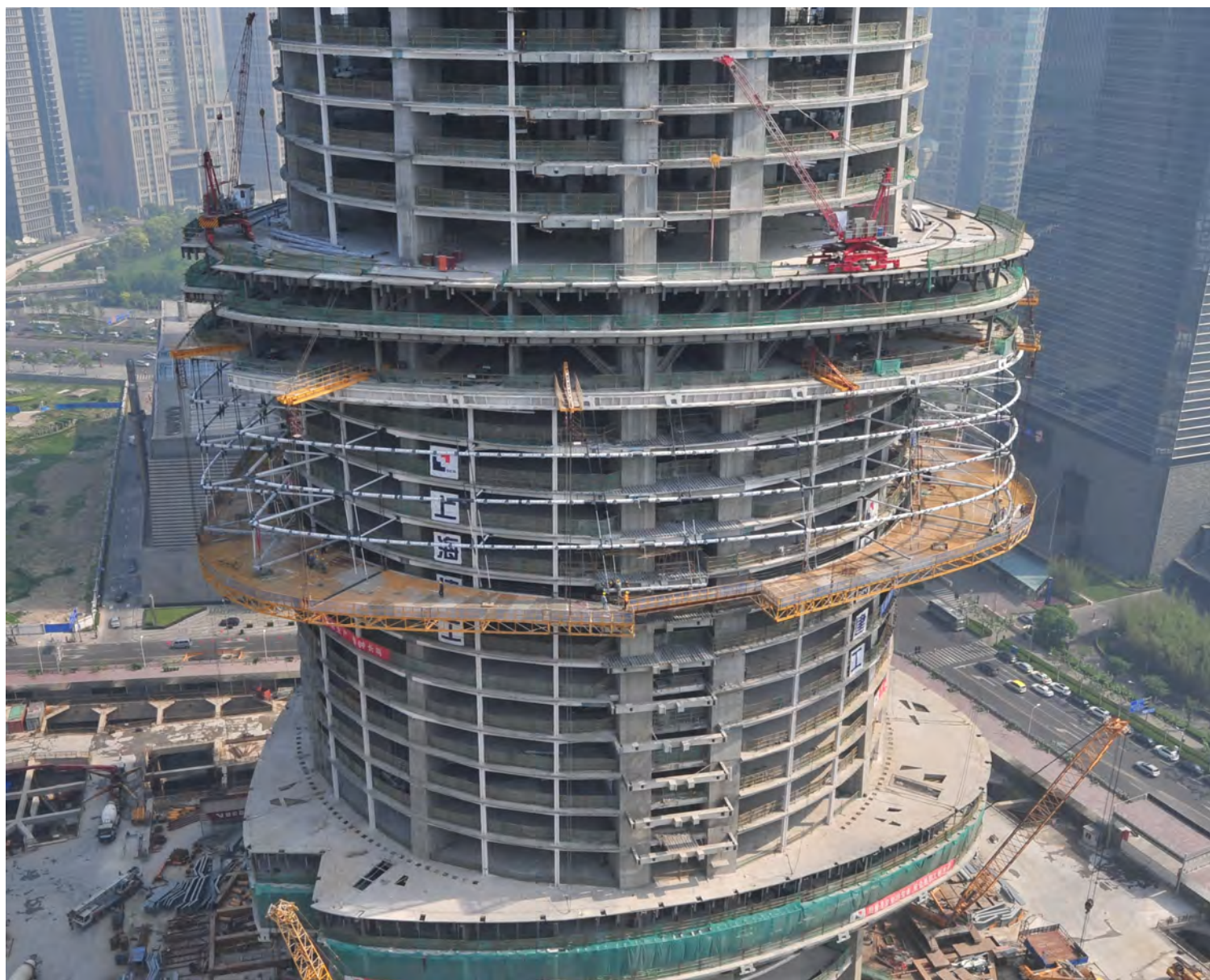
Figure 5.12. The walking tower crane and overall lift platform system (Source: Shanghai Construction Group) 图5.12. 行走式小塔吊和整体升降平台 (来源: 上海建工集团)
