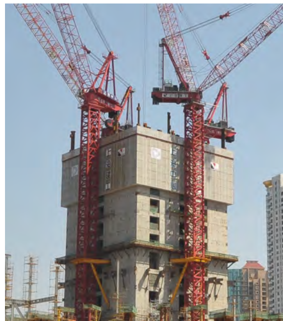
Figure 5.10. Hydraulic jack-up steel platform and template scaffold system (Source: Shanghai Construction Group)
