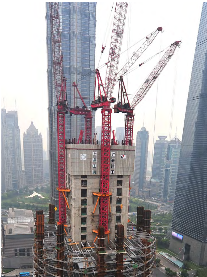
Figure 5.11. Four heavy cranes arranged in the way of out-door hanging (Source: Shanghai Construction Group)
