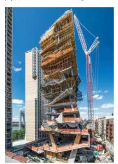
Figure 6. Cascade reshoring during construction (Source: Matthew Melrose)
