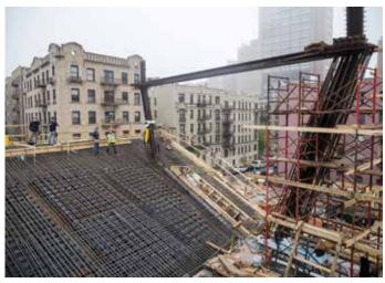
Figure 14. Combination of state-of-the-art materials and technology: void formers, high strength rebar, high strength concrete, and structural steel embedded in columns form the Auditorium structure at the base of the Cascade (Source: Matthew Melrose)
