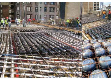
Figure 7. Construction materials: slab void formers placed between bands of bonded post-tensioning (Source: Matthew Melrose)
