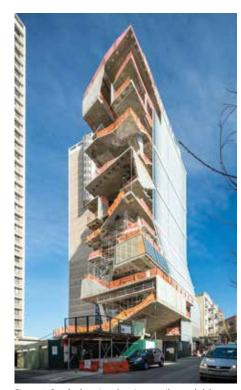
Figure 4. South elevation showing cantilevered slabs with varying floor-to-floor slab edge positions (Source: Matthew Melrose)
