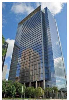
Figure 4. PVDF liquid exterior coating on the Hess Tower in Houston, Texas (Source: AkzoNobel)
