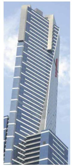
Figure 10. The Eureka Tower is a powder coated 975foot skyscraper located in the Southbank precinct of Melbourne, Victoria (Source: AkzoNobel)
