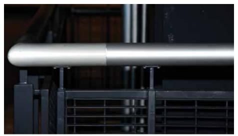
Figure 11. Naturally occurring color variations in newly installed anodized aluminum (Source: AkzoNobel)
