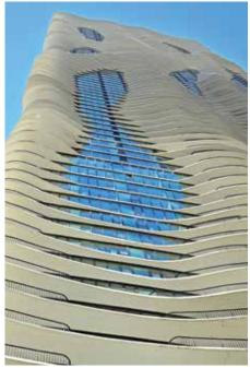
Figure 3. PVDF liquid exterior coating on the Aqua Tower in downtown Chicago. Designed by Jeanne Gang, Aqua is the tallest built skyscraper to be designed by a female architect (Source: AkzoNobel)
