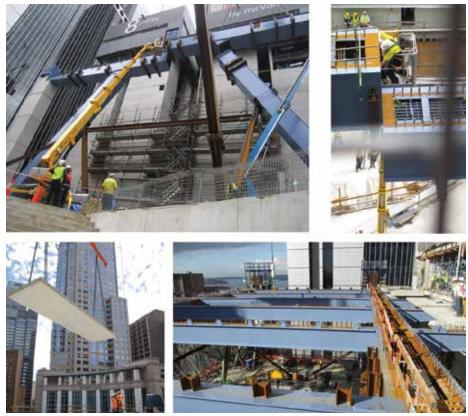
Figure 10. Composite megaframe assembly (Source: Arup)
