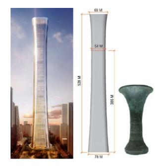
**Figure 1.** Rendering elevation view and the size of "Zun" (© Kohn Pedersen Fox Associates).
