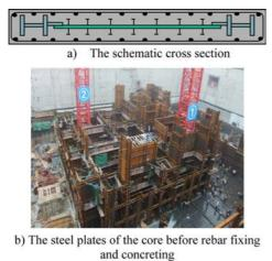
Figure 7. The Composite shear wall.
