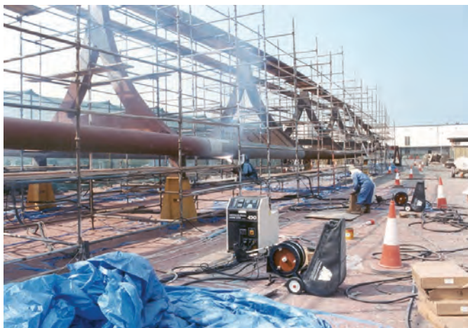
Figure 6. Arc spray and paint application ongoing at yard (Source: Jotun) 图6. 外骨架钢结构在工厂车间施工电弧喷铝和油漆施工 (来源: 佐敦)
