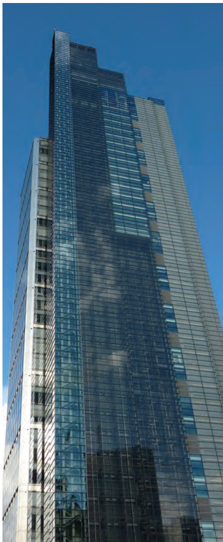
Figure 1. Heron Tower, London. South-facing photovoltaic integrated façade generating 2.5% of building electricity (Source: Philip Oldfield) 图1. 伦敦的苍鹭大厦。朝南的光伏立面满足了建筑2.5%的电能需求（来源：Philip Oldfield）
