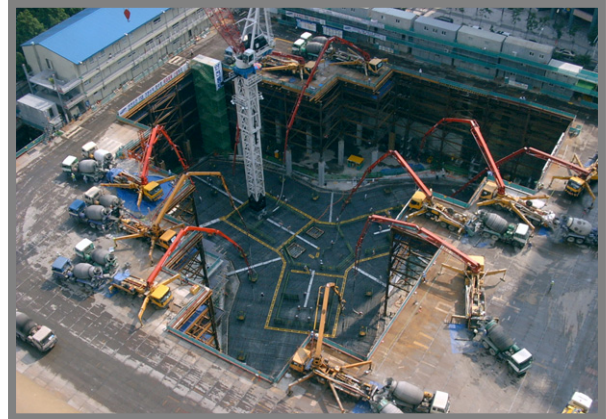
Figure 8: Casting the foundation mat
