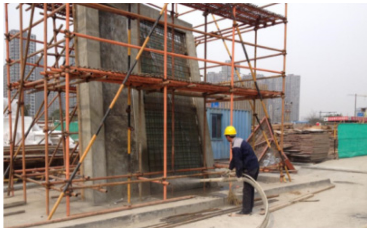
(a) Shot-concrete on backing structures
