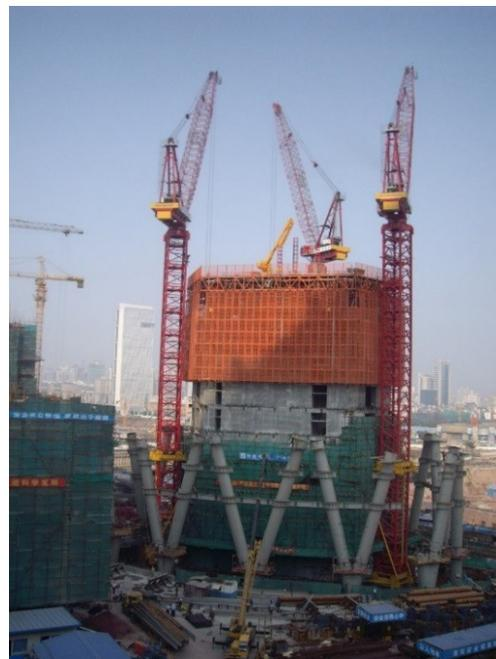
**Figure 44.** Climb-form system of central core.
