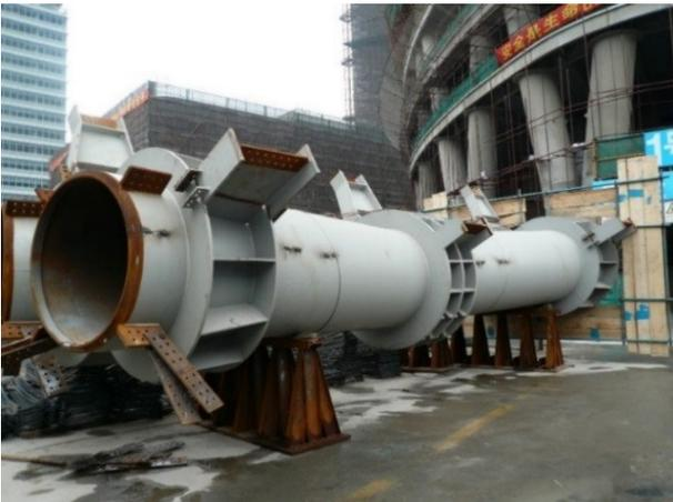
**Figure 45.** Prefabricated diagrid steelwork.
