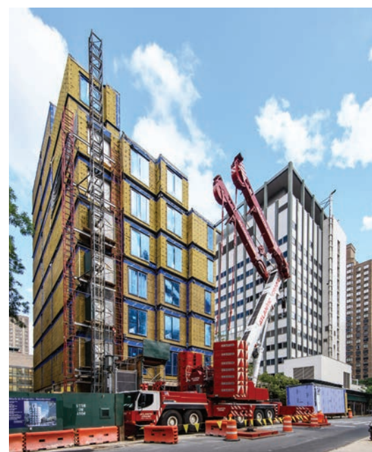
Figure 4. Modular assembly underway at Carmel Place.
