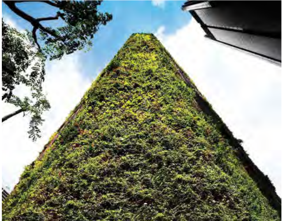
Figure 11. Creeper vines, planted in 1,800 fiberglass planters along the building's exterior, have grown steadily over less than two years, covering several of its surfaces. © Patrick Bingham-Hall
