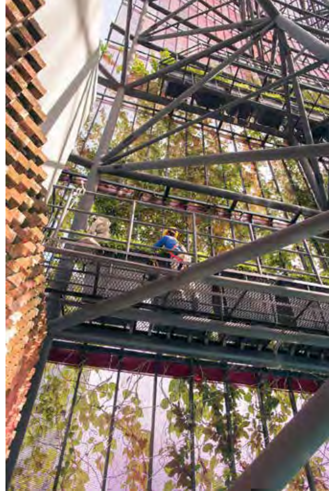
Figure 13. The façade structure consists of a maintenance catwalk, fiberglass planters and an expanded mesh screen.
