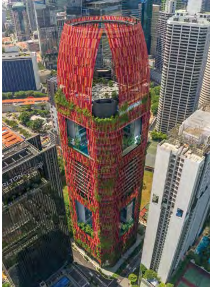
Figure 10. Oasia's open-sided, cross-ventilated breezeway atria contrast with the hermetically sealed towers in the immediate neighborhood. © K Kopter
