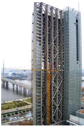
Figure 5e. Outrigger truss detail
