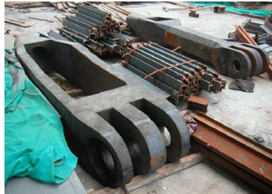
Figure 4n. Rocker clevis castings on site
