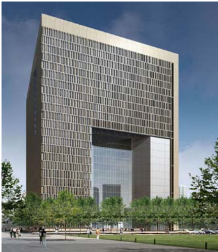
Figure 4c. Vierendeel bridge at south façade
