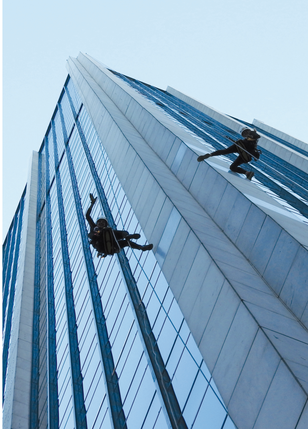
Figure 1. Julie Foster (left) and Amy DeLuca (right) performing a façade inspection. © Henry Marksbury
