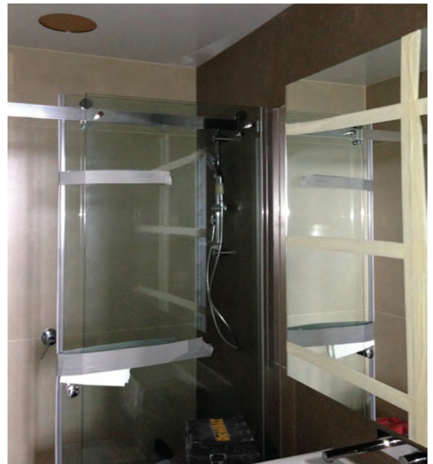
Figure 1. Prefabricated Prefinished Volumetric Construction (PPVC) of bathroom pods in an Australian tall building (left) installed on the floor during construction, with pre-finished interior (right). © G. Marfella
