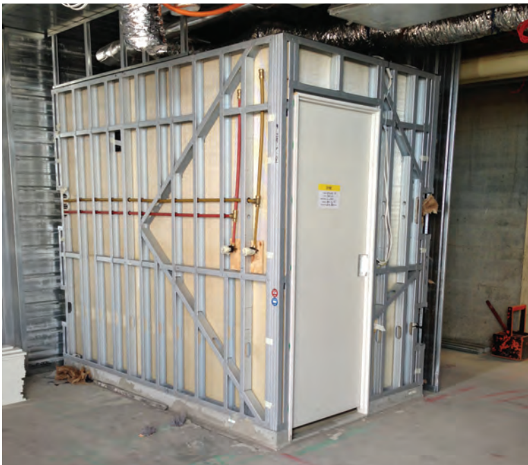
Figure 1. Prefabricated Prefinished Volumetric Construction (PPVC) of bathroom pods in an Australian tall building (left) installed on the floor during construction, with pre-finished interior (right). © G. Marfella
