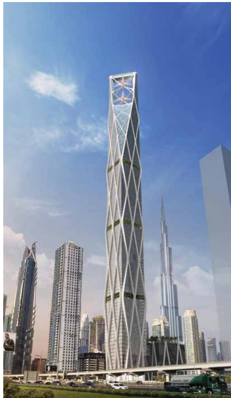
Figure 5. SRG Tower, Dubai—an example of building shaping being used to reduce response. © Killa Design
