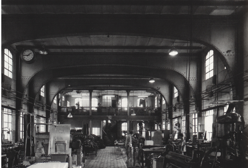
Figure 14. Jules Saulnier and Armand Moisant, Menier Chocolate Factory, Noisel, 1869. Interior showing iron structure with portal bracing.(Unknown source.)
