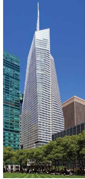
Figure 14. The high-performance curtain wall of Bank of America Tower, New York City, minimizes solar heat gain through low-e glass and a heat-reflecting ceramic frit. © Marshall Gerometta
