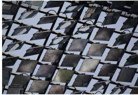
Figure 3. The heliostats on One Central Park, Sydney, provide hours of sunlight and heating to areas normally shaded. © Terri Meyer Boake
