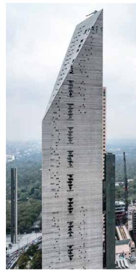
Figure 6. Torre Reforma, Mexico City, uses its concrete shear walls to limit solar heat gain.  $\ensuremath{\mathbb{S}}$  HEXA
