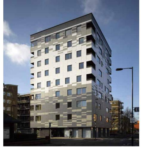
Figure 12. Completed in 2009, Stadthaus, London, was one of the first modern tall buildings to use cross-laminated timber (CLT) panels. © Will Pryce
