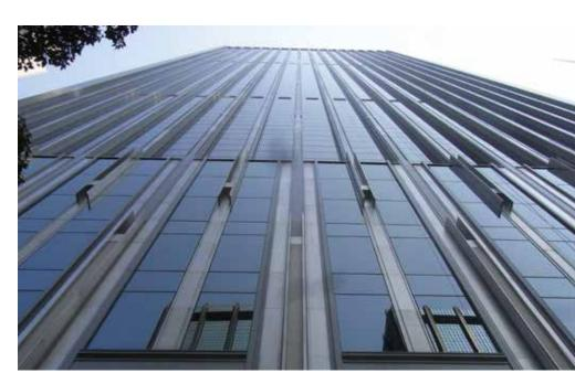
Figure 11. A façade detail view of China Resources Building, Hong Kong, which features a special low-e coating to limit solar gain. © Powfreytmn (cc by-sa)
