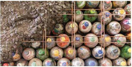
Figure 5. In this configuration, ecobricks purely fill a void, as the surrounding concrete provides overall support. A reference-193 (1.93 kg/m2) steel mesh was placed on top of the ecobricks to hold them in position, preventing them from moving when concrete was poured, and to control and limit surface cracking.
