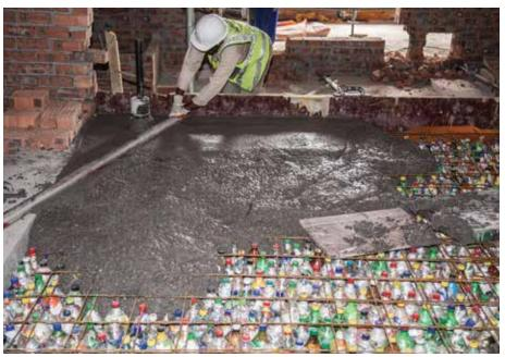
Figure 2. Ecobricks as void formers being filled with concrete in non-load-bearing areas of the floor at the Ridge where no services are required.
