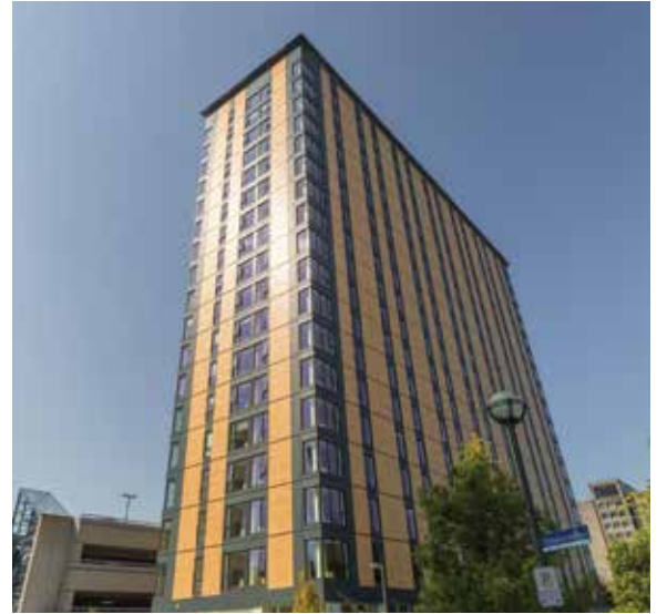
Figure 1. Brock Commons Tallwood House, University of British Columbia, Vancouver, 18 stories, 2017, under construction at left, and completed at right, uses a reinforced-concrete core and timber gravity-resisting system. © Brudder, courtesy of naturallywood.com
