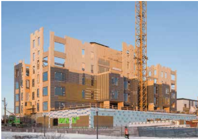
Figure 2. Origine, Quebec City, Canada, under construction at left, and completed at right, uses 12 stories of mass timber on top of a one-story concrete podium. © Nordic Structures/Stephane Groleau
