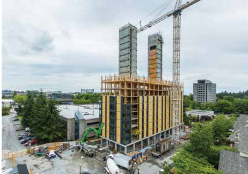
Figure 1. Brock Commons Tallwood House, University of British Columbia, Vancouver, 18 stories, 2017, under construction at left, and completed at right, uses a reinforced-concrete core and timber gravity-resisting system. © Brudder, courtesy of naturallywood.com
