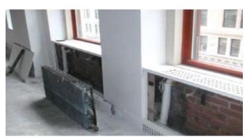
Installing insulated reflective barriers behind radiator units on the perimeter of the Empire State building
