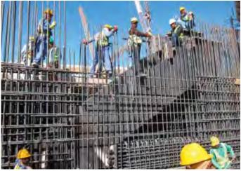
Figure 8. Mega link beam during installation. 图8. 在安装中的巨型连梁
