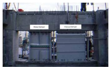
Figure 4. A Viscous Damper and a Brake Damper (Source : Toranomon-Roppongi Work Office)
