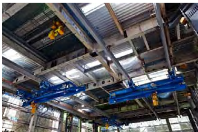
Figure 9. The utilization of the existing roof structure (source:TAISEI Corp.)
