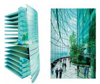
Figure 8. The buffer space in Shanghai tower (Source: http://openingbuilding.com) 图8. 上海中心缓冲空间 (资料来源: http://openingbuilding.com)
