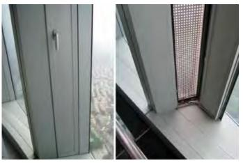
Figure 6. The details of operable walls in Zifeng Tower (Source: Jianqiang li) 图6. 紫峰大厦中可开启的外墙细部 (资料来源: 李建强)
