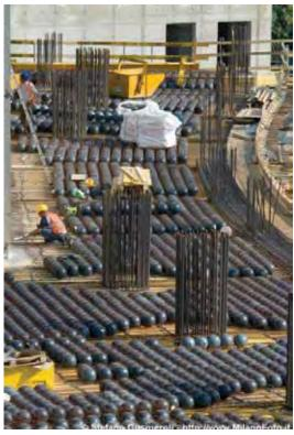
Figure 2. "Bubbledeck" technology. This elements allow a 20% concrete saving if compared to standard solutions. (Source: courtesy of Cobiax) 图2. "泡沫板"技术。此元素可比标准方案节省20%的混凝土。(来源:由 Cobiax提供的照片)
