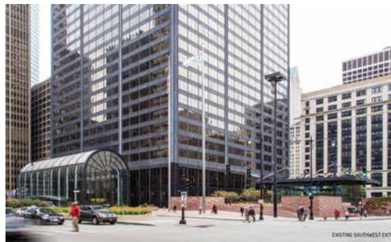
Figure 10. The existing southwest corner view from Wacker and Jackson, before construction began on the new podium. The 1985 "Lunchbox" (left) and 1993 Skydeck entrance pavilion (right) can be seen. © Gensler
