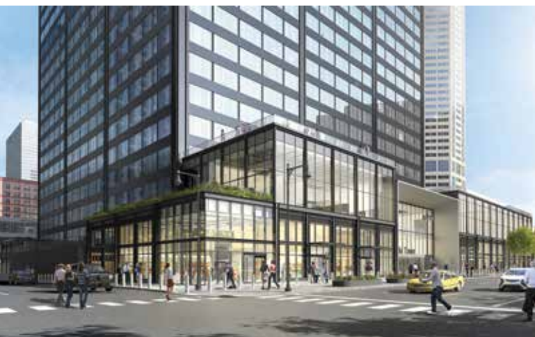
Figure 9. New northwest corner view from Wacker and Adams. The new Wacker Lobby entrance is clad in custom white terra-cotta panels. Image courtesy of Blackstone
