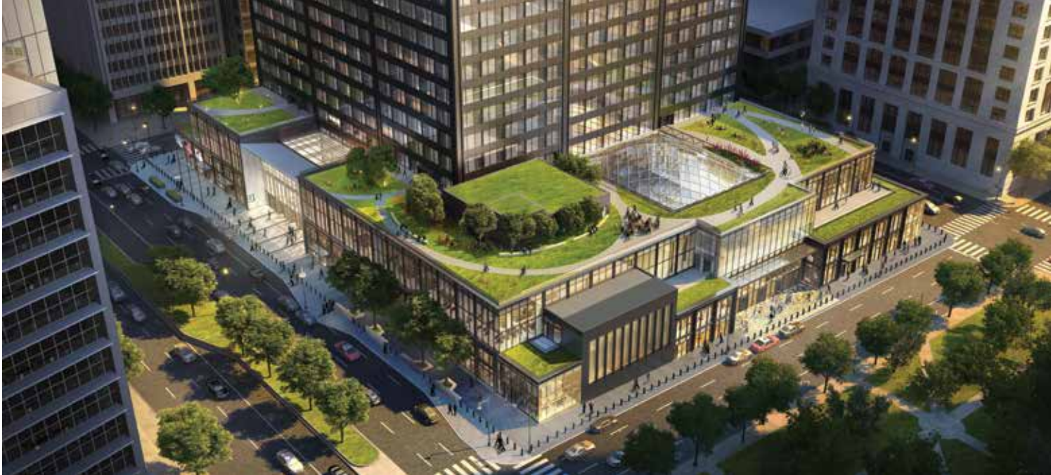
Figure 1. Aerial view of Catalog, the new retail podium of the Willis Tower, from the southwest. Image courtesy of Blackstone
