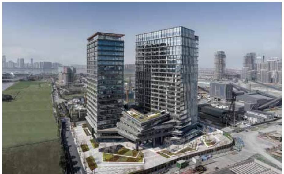
Figure 7. Aoti Vanke Centre in Hangzhou disrupts the established norm in office architecture by featuring a courtyard garden in the central core.
