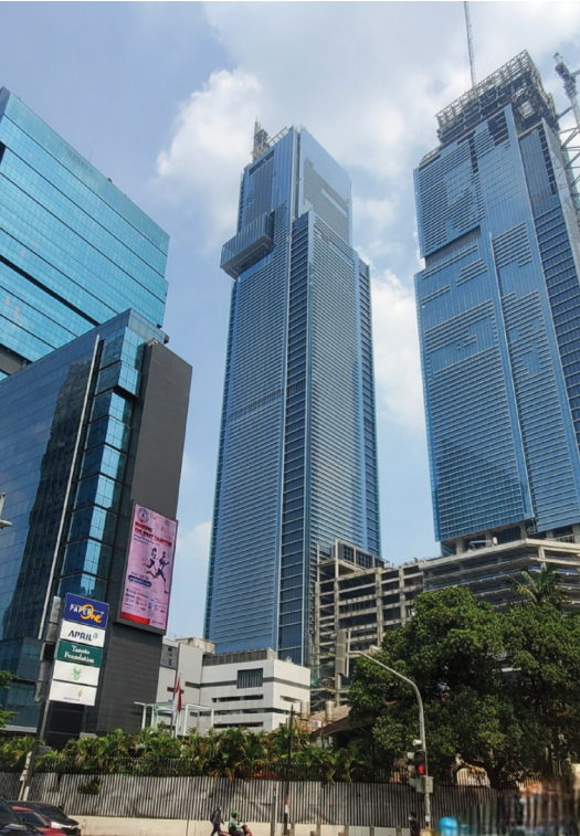
Figure 13. The Autograph Tower, Jakarta, at 383 meters, is now the tallest building in Indonesia. © Tansri Muliani
