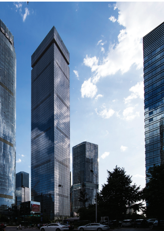
Figure 15. Glory · Xi'an International Finance Center, Xi'an, entered the list of the World's 100 Tallest Buildings in 2022 at 350 meters. © Beijing Institute of Architectural Design
