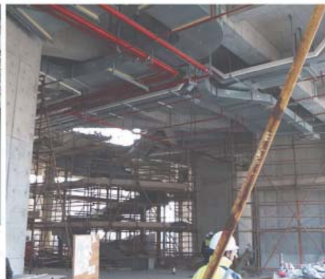
From the Site Installation
