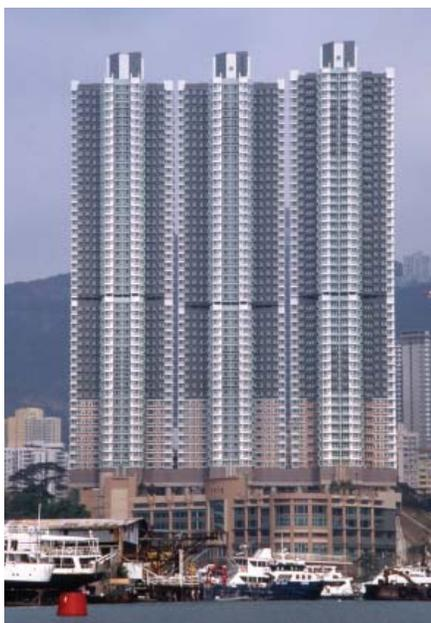
Figure 4. Hong Kong: the presence of common-level “refuge floors” in many of the separate towers allow easy incorporation of short skybridge linkages © Antony Wood
