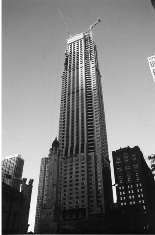
Figure 2 Photo of the Park Tower under construction.
