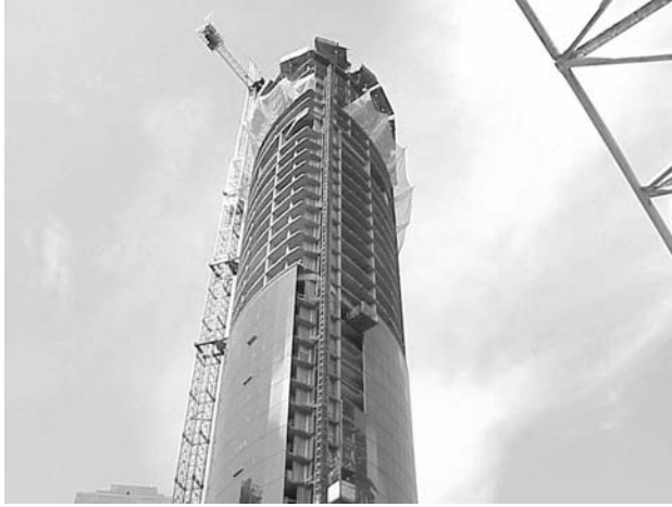
Figure 5 Wall Centre under construction.
