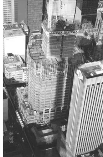
Changes to the requirements for formwork caused an increase in the cost of conventional systems such as table forms that would have normally been adopted for this type of floor. Various alternatives were considered before adopting a metal decking system as permanent formwork for the slabs. This reduction in conventional formwork meant that a 4-day floor cycle could be achieved with resulting benefits in construction time.
