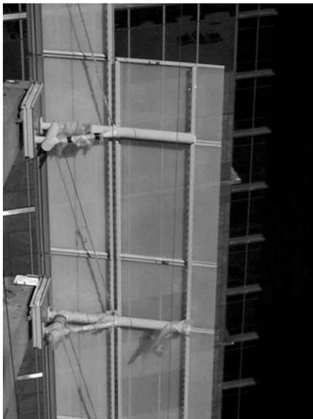
**Figure 25** Façade fin cantilevered steel framing.
