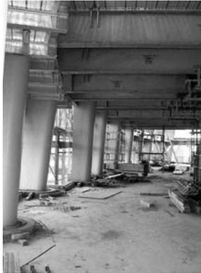
**Figure 5** Level 42 plantroom needle columns and steel framing.
