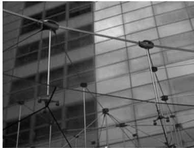
**Figure 32** Piazza canopy spider and hanger connections.
