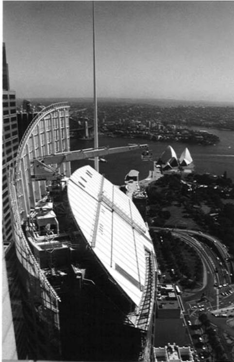
**Figure 33** Aerial view of BMU and sloping roof.
