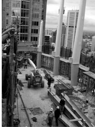
**Figure 29** West sail needle erection.
