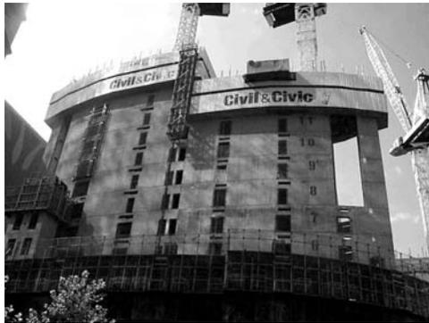
**Figure 7** Core jumpform construction.
