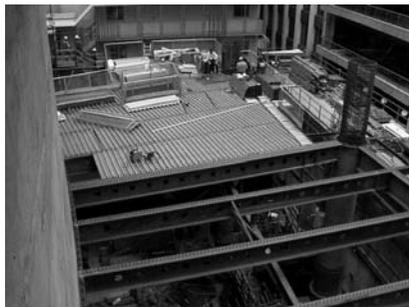
**Figure 12** Accelerated Level 3 structural steel framing.
