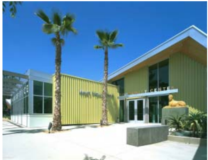
West Hollywood Community Center Hollywood, California
