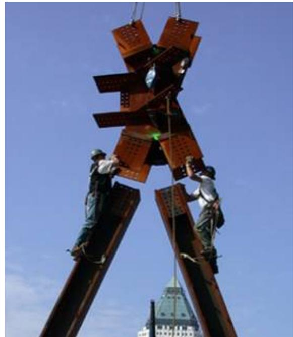
Figure 11. Installation of 6 ton node connector
