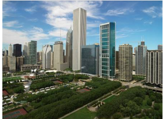
Figure 2. Aerial view of site, with the finished building right of center (photo courtesy SCB)
