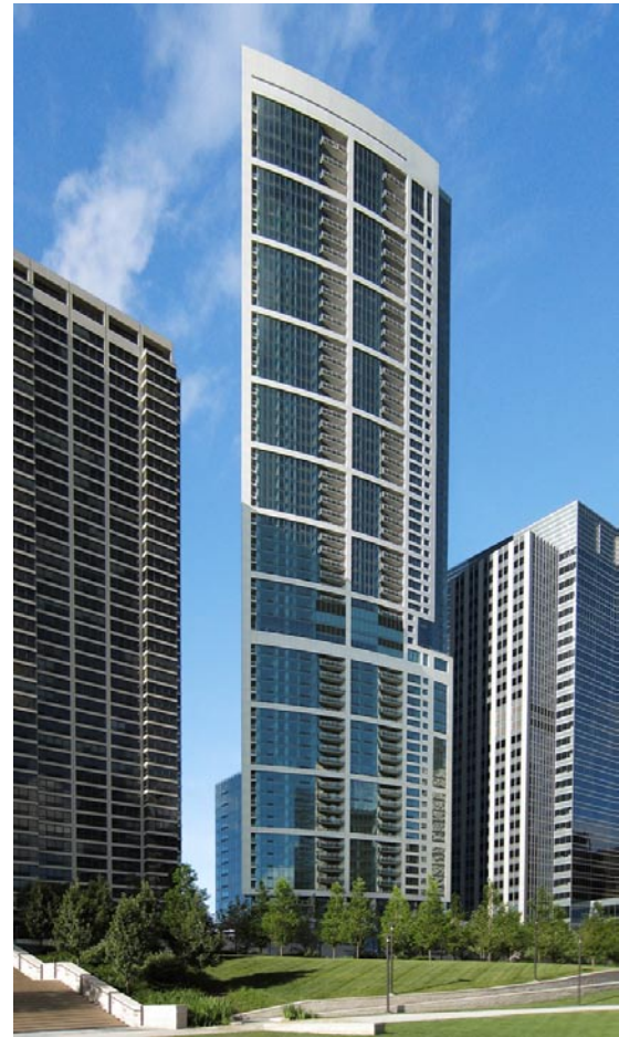
Figure 5. North façade (photo courtesy SCB)
