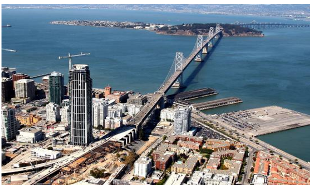
Figure 11. Aerial view of construction site (photo courtesy MKA)
