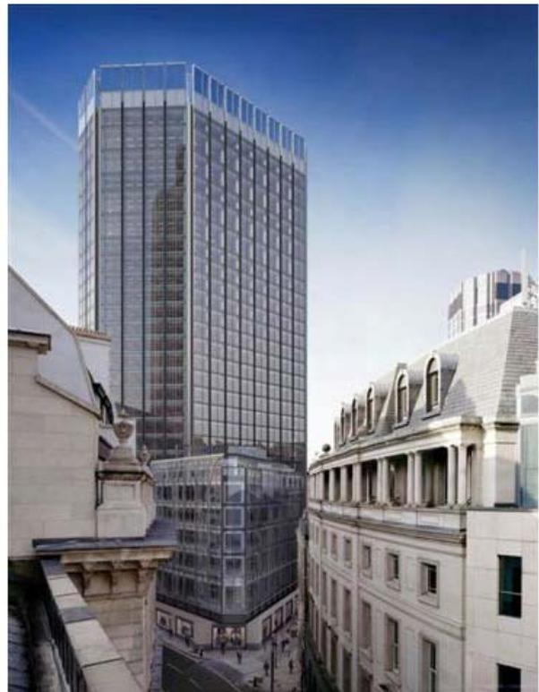
Figure 11. Originally completed in 1970, the former London Stock Exchange Tower has been renovated and reclad in glass - a design by Nicholas Grimshaw Architects. (Source Nicholas Grimshaw Architects)
