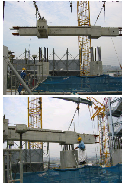
Photo 1. The pre-cast beam unit through column method of construction
