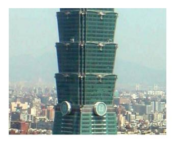
**Fig. 3.** A close-up of the tower corner clearly shows the 'sawtooth' treatment above Floor 25 for wind vortex reduction.
