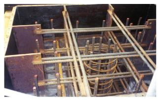
**Fig. 8.** Concrete fill is reinforced by vertical bars threaded through diaphragm holes and a spiral-wrapped core threaded through the central manhole.
