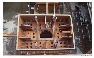
**Fig. 6.** A supercolumn box just below its field splice location. High strength concrete enters through the pipe at right to fill the box from bottom up in two-story lifts.
