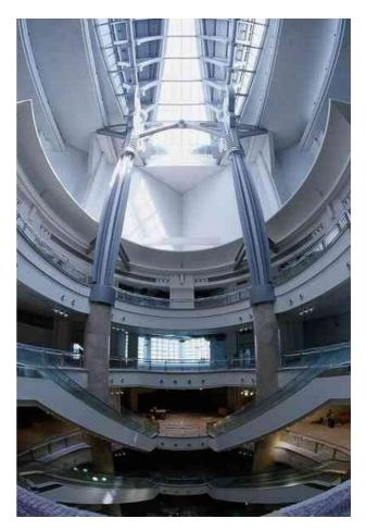
**Fig. 12.** Twin Vierendeel trusses span the shopping mall atrium within the building podium.
