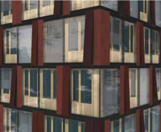
Figure 11. The opaque façade area can be used to accommodate structural elements. © CREE/Architekten Hermann Kaufmann
