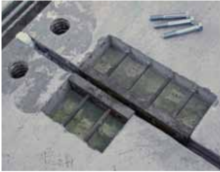
Figure 7. Integrated connections in prefabricated panels.
