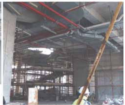
From the Site Installation
