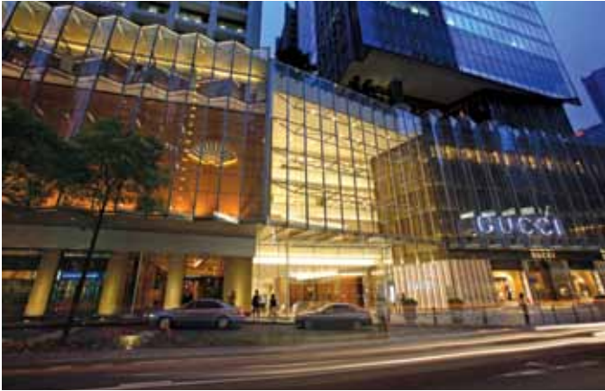
Figure 3. The Landmark, Hong Kong. © Hongkong Land
